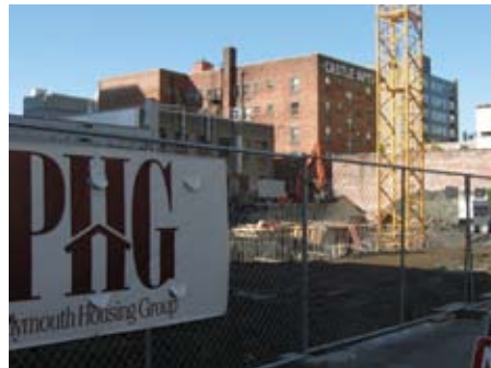
Above: the construction site at 3rd & Blanchard
