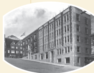
Plymouth's renovation of the Pacific Hotel wins National Historic Preservation award.
