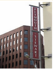
Plymouth renovates the old St. Regis Hotel in 2006 and renames it Plymouth on Stewart.
