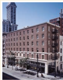
The historic St. Charles Hotel was remodeled in 2004.
